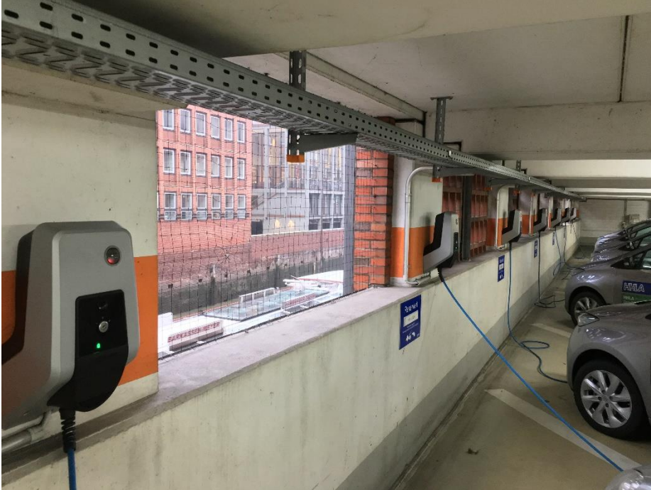
Parking garage Hamburg warehouse district
